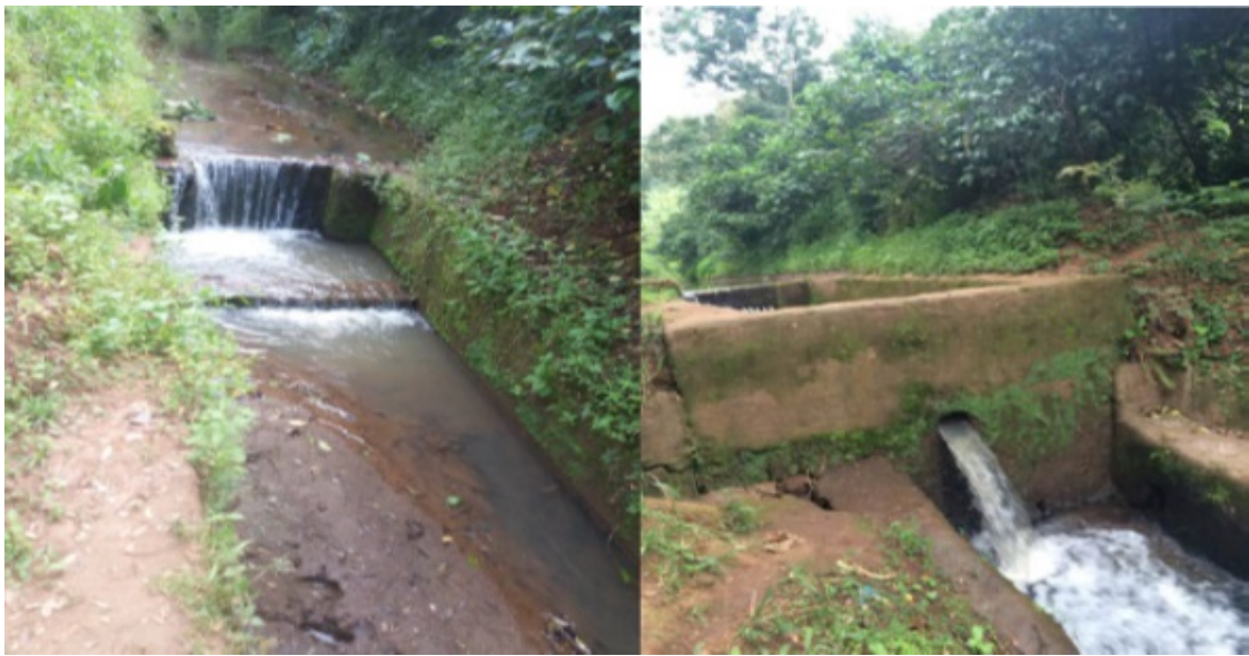
Figure 1 Dilla Town Water Treatment Plant Aeration System
