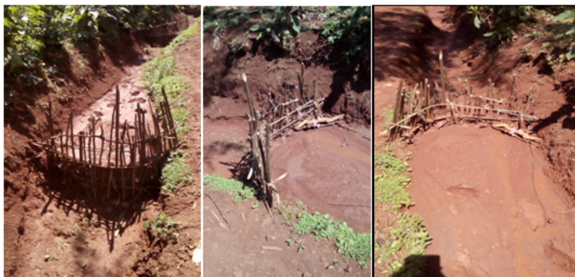
Figure 5. Wooden check dams made by the local farmers (Wonago area). Source: Haile, 2017
